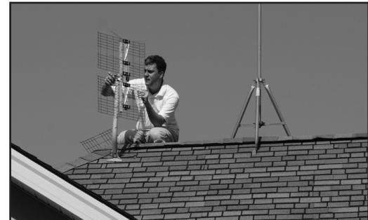
If your signal is weak, check the length of your cable run (the shorter the better) and remove any splitters or diplexers. Check all connectors/junctions for secure fit or corrosion. If your cable run must be longer than 75 feet, or you must use a splitter, consider a pre-amplifier-- [http://www.antennasdirect.com/antenna\\_amplifier.html](http://www.antennasdirect.com/antenna_amplifier.html).
